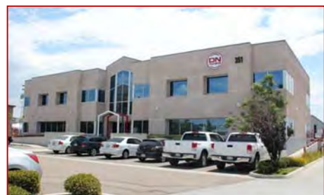
Local DN Tanks' headquarters located in El Cajon, CA
